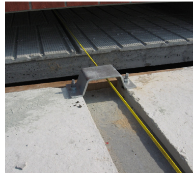
Stop attached to concrete floor
